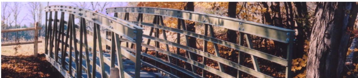
40' x 6' Footbridge on the McDade Trail - Delaware Water Gap
